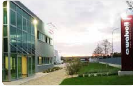
Business Unit Hydrocontrol Castel San Pietro (BO) • Italy
